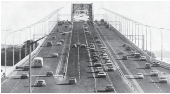
**Before-** Half of the bridge was 50 years old and required complete rebuilding, and would remain closed for the duration of the project. A buffer zone was striped on the available bridge span during Phase 1 of construction. Lane delineators were used to create one lane in each direction. The result was massive traffic queues up to 6 miles (10 km) on Fridays and Sundays. A new solution was necessary.
